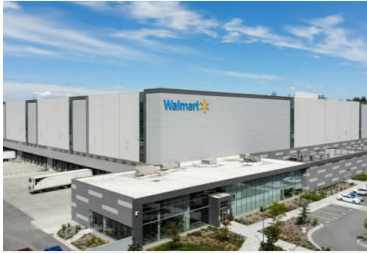
Walmart Distribution Center Automation & Expansion
